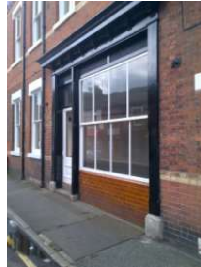
A modern timber shop front, traditionally designed with ceramic brick stall riser.
