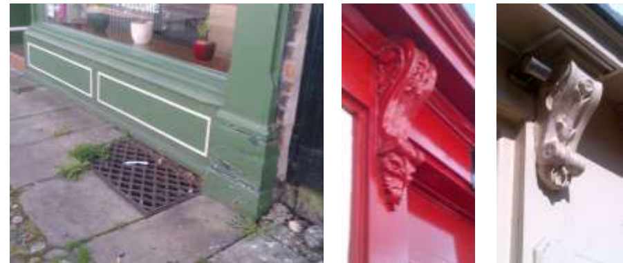
Traditional shop front components – stallriser and corbel brackets
